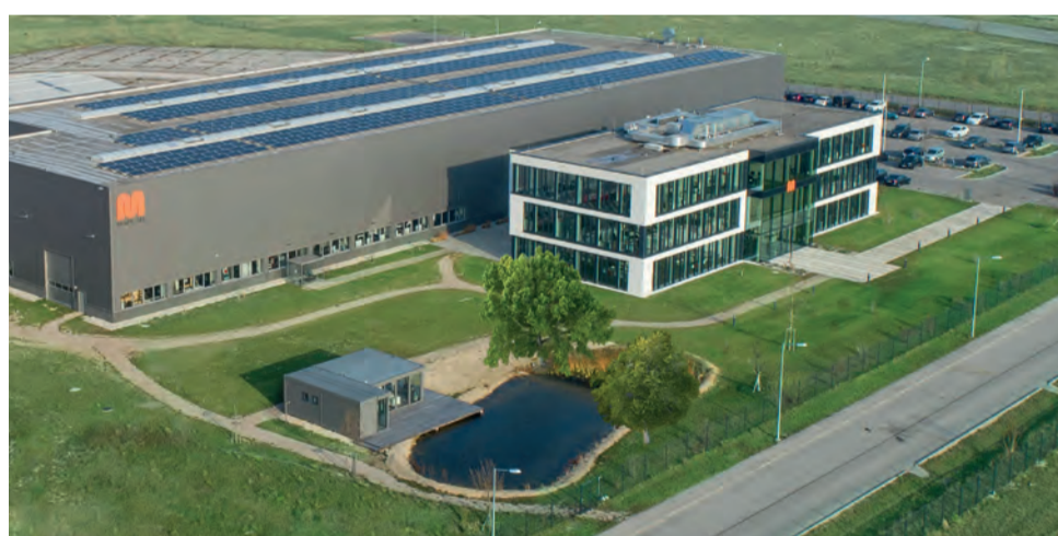
Operational Excellence from the Top: Kottlingbrunn headquarters with the fire protection pond and a glass bungalow for meetings.
